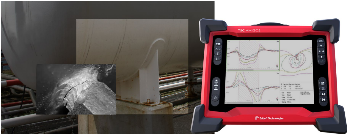
Figure 15 Saddle weld inspection with Amigo2 ACFM
